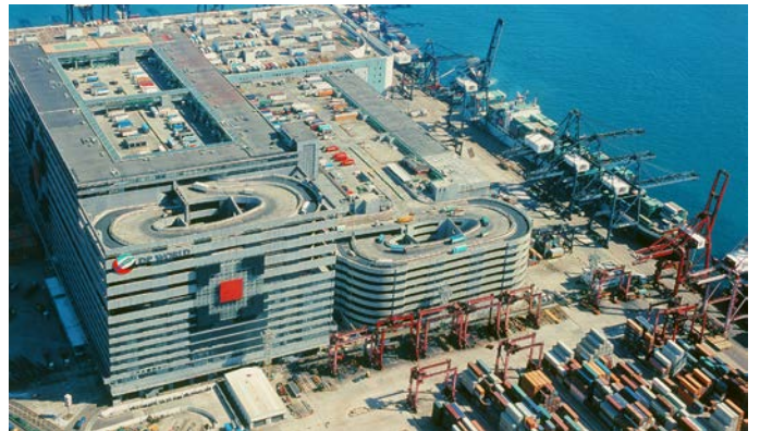
Cargo services headquarters - Hong Kong
